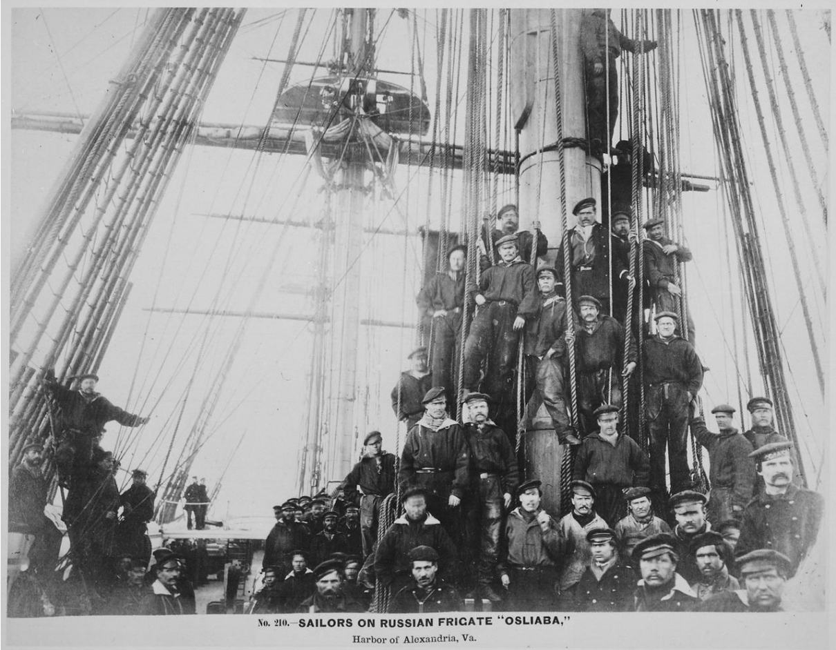
Figure 15 - Running rigging and shrouds "Hawser-Laid", right-handed. Russian frigate, Osliba, ca. 1863.
